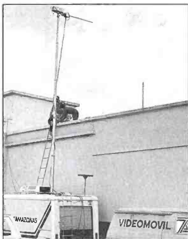
Setting up at the soccer stadium for microwave transmission. On most remotes such as soccer matches, set-up takes 30 minutes or less.
